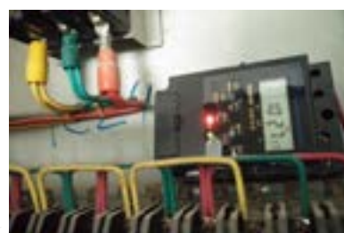
◆ Installation time controller
