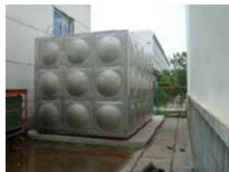
◆ Hot water storage tank
